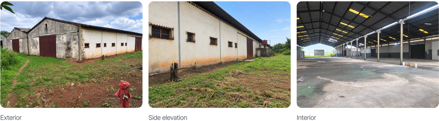
Figure 3. The warehouse today. Exterior, side elevation, and interior of the building before retrofit.
